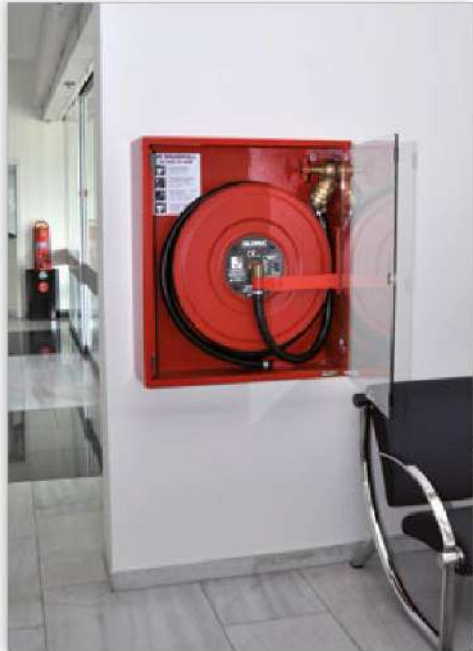
GLORIA wall hydrant with semi-rigid hose and glass door.
